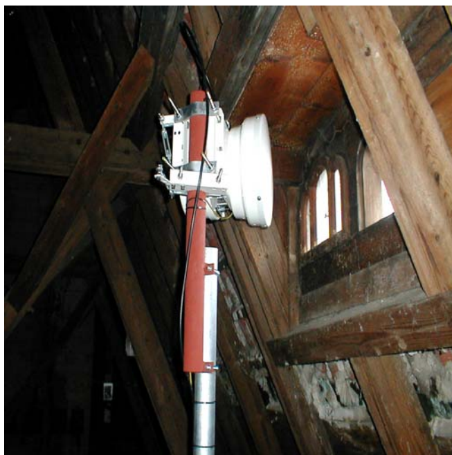
Obr.2 Parabola RR spoja – KC Smolenice
