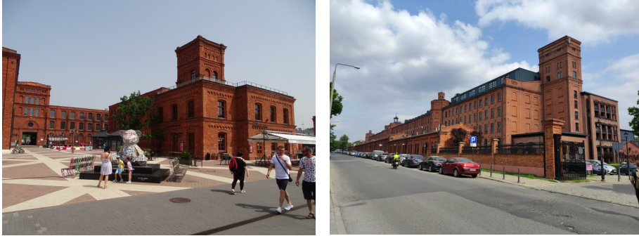
Fig. 3. Manufaktura shopping centre (former Israel Poznansky factory) and Scheibler Lofts residential complex
