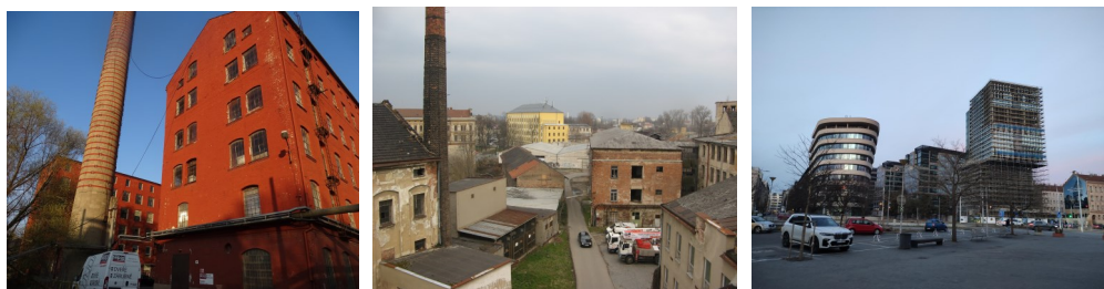
Fig. 4. Former textile factories (Mosilana, Vlněna) and construction of a new office and residential complex (Nová Vlněna)
