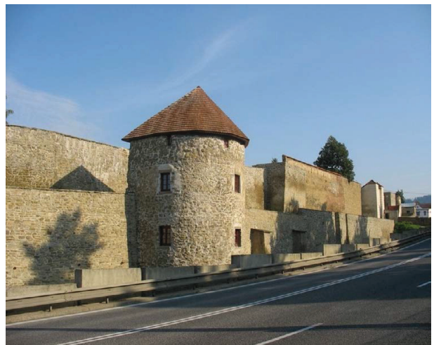
Fig. 1: Levoča city fortifications, view from the east. Photo: Levoča Information Office.
