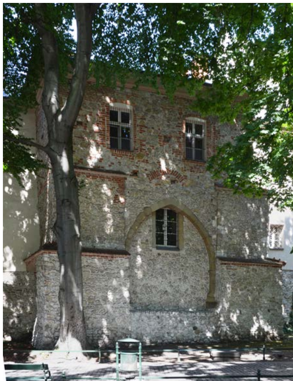
Fig. 15: Cracow, the barbican of the new Butchers' Gate. Photo: Piotr Pajor.
