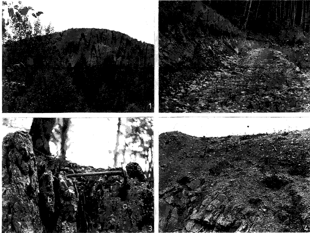
Plate 1: Fig. 1 - cutting on a forest road in the Svinské Chlievy massif, at the locality of the Svinské Chlievy Formation (uppermost Paleocene - Lower Eocene). Fig. 2 - cutting on a forest road, Svinské Chlievy. Transgressive base (a) of the Svinské Chlievy formation (4 m) (in the basement are Wetterstein limestones), above are conglomerates with three deposits of red clays. Fig. 3 - vertically erected horizon of Malenica onyxites: a-underlying, b-overlying Súfov conglomerates. Fig. 4 - transgression of Lutetian conglomerates on Upper Triassic dolomites of the Strážov Unit. Quarry at Malá Čierna.
