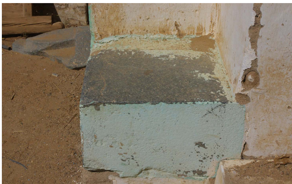
Hudec, Fig. 2. Dressed black granite blocks in front of the entrance to the old mosque in 2017 (Photo: Jozef Hudec)
