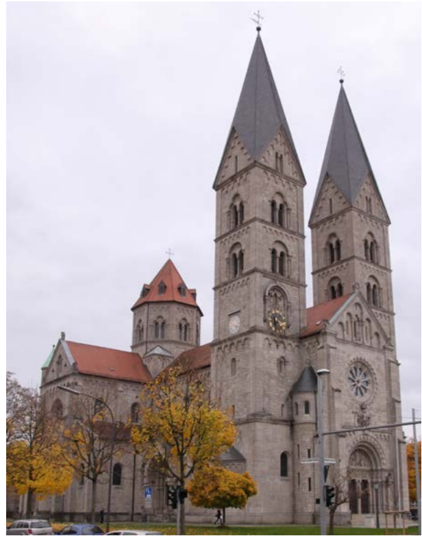
Fig. 5. Würzburg, St. Adalbero's Church [ Adalberokirche ], 1894–1899, façade. Photo by author, 2010.
