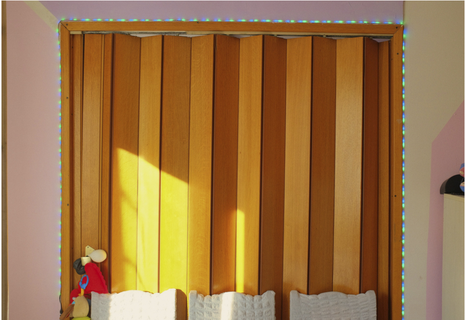
Figure 4: Improvised wooden partition made from closed accordion doors, repurposed as a permanent wall between rooms and outlined with LED lights. Author: Sara Nikolić (2024).
