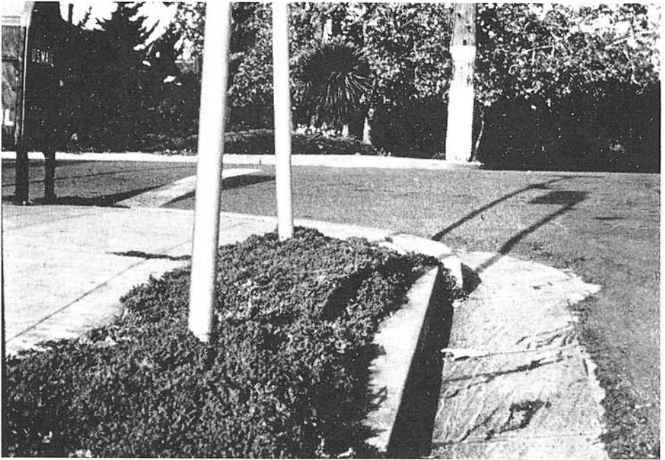
Fig. 4. Damage to a curb in the city of Hayward due to right-lateral tectonic creep along the Hayward fault.
