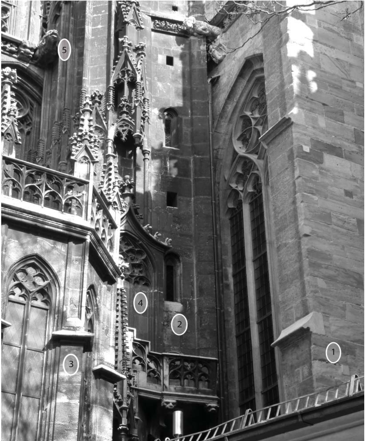
Fig. 4. South tower, north-east corner and junction with choir (looking north-west) showing: 1: choir; 2: staircase turret; 3: chapel of St. Catherine; 4: buttress; 5: gargoyle. Photo: T. Jukes
