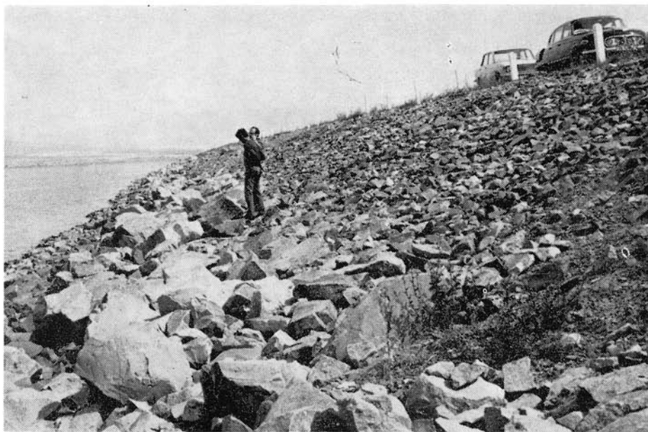
Fig. 10. Unsorted boulders of propylitized andesite in the rip-rap of the earth dam of the East Slovakian water reservoir. The intense disintegration of andesite by its weathering is seen on the right side of the photography. Big bloks in the lower part were brought in only during the reconstruction of the rip-rap.
