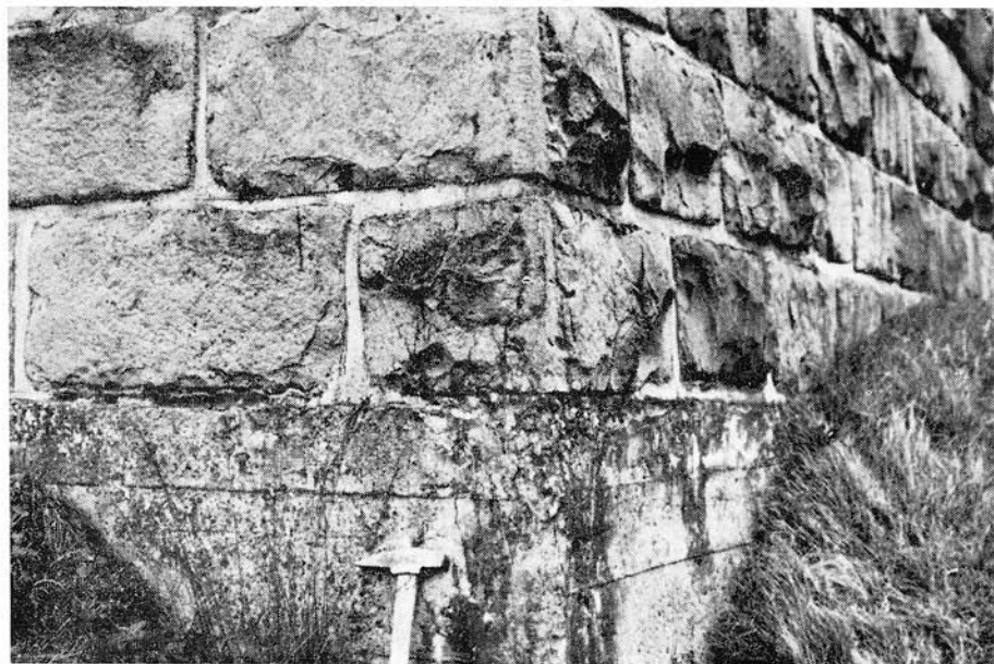
Fig. 14. Rupture of the ashlar stones and concrete by the action of capillary suction of water and its freezing in the surficial part of the ashlar stones and concrete in the lower portion of the pier wall.
