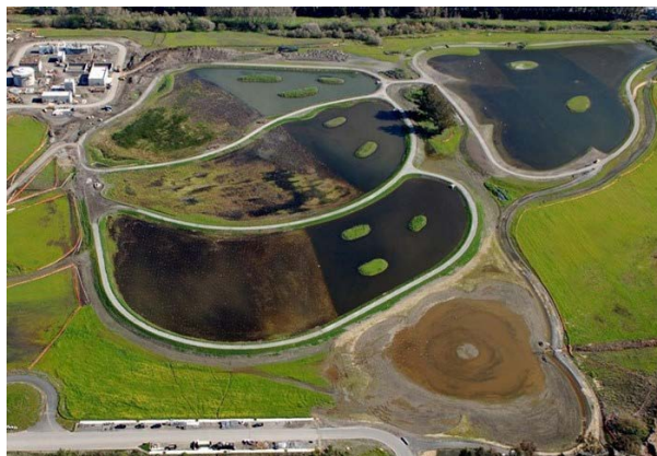
Obr. 1: Patricia Jobanson & Carollo Engineers: Petaluma Wetlands Park and Ellis Creek Water Recycling Facility (2001–2009), Petaluma, California. Zdroj: https://lancasteronline.com/features/home_garden/boating-in-a-sewage-treatment-plant-how-this-artist-designs-inviting-and-functional-landscapes/article_26ff3952-83ed-11e5-b700-a710cdebfd1b0.html
