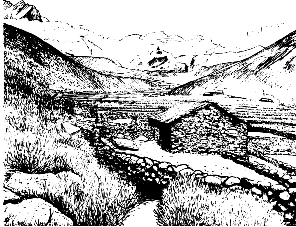
Fig. 16. Stone walls of the seasonal Sherpa village of Dingpocche (4 200 m a.s.l.) south of the Chomolongma Massif are built of blocks of paragneisses, phylites and granites of fluvio-glacial and slope accumulations
