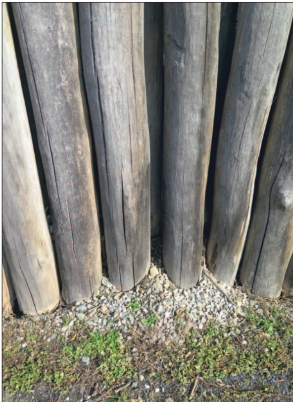
Fig. 4. Modrá. Oak poles of the palisade embedded in crushed stones.
