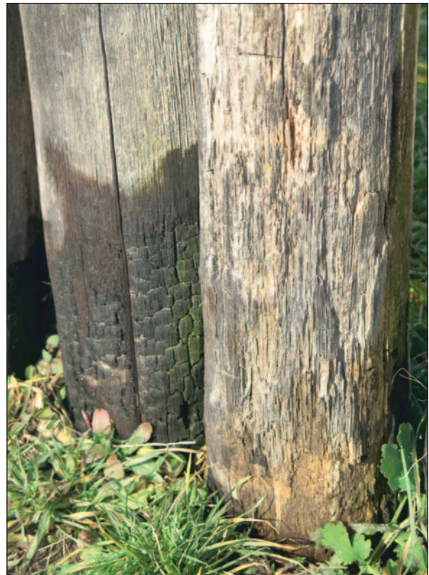
Fig. 5. Modrá. Oak poles of the palisade: on the left well charred, on the right improperly charred.
