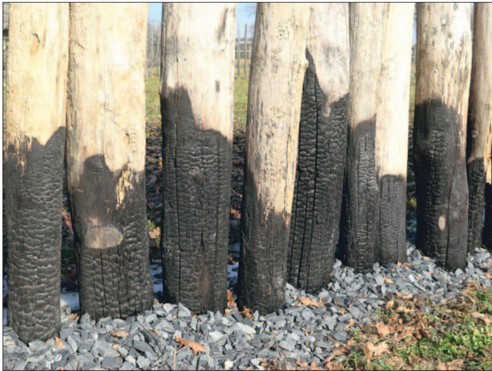
Fig. 7. Modrá. Well charred lower parts of an oak pole.
