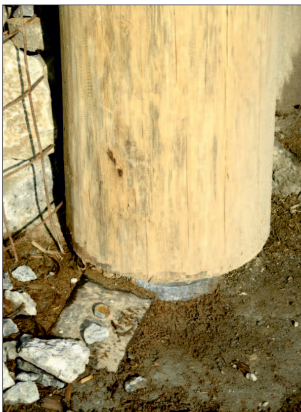
Fig. 17. Modrá. Details of the lower part of a red spruce pole from the gate construction on a lead pad.
