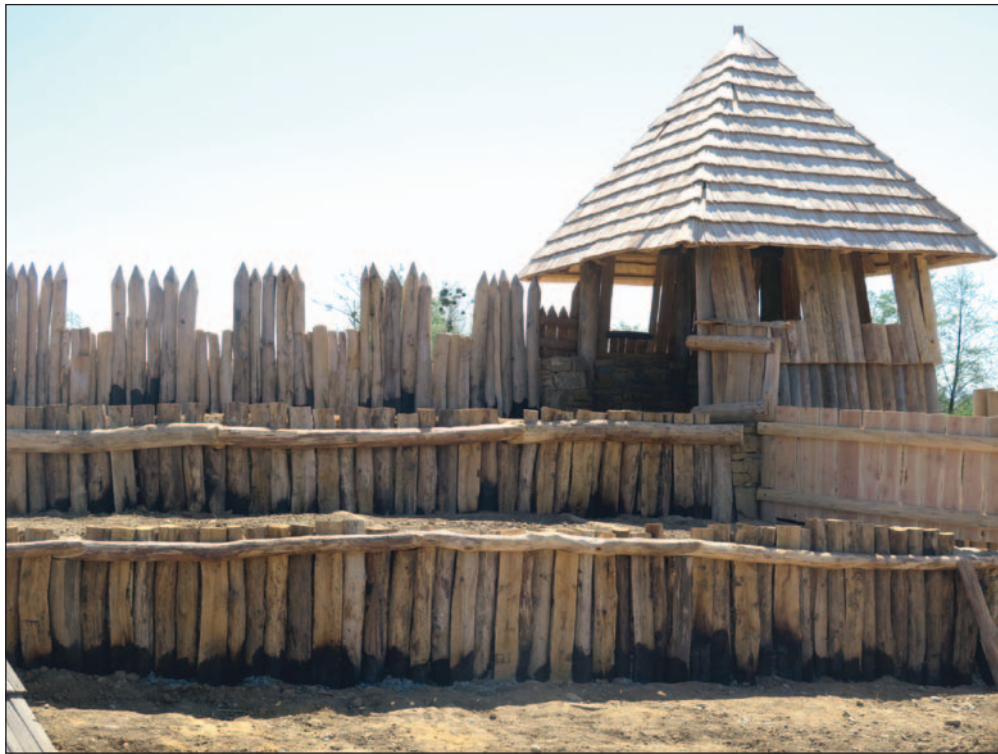
Fig. 16. Modrá. The stepped body of the wooden-soil construction of the fortifications and the defensive tower, back view.
