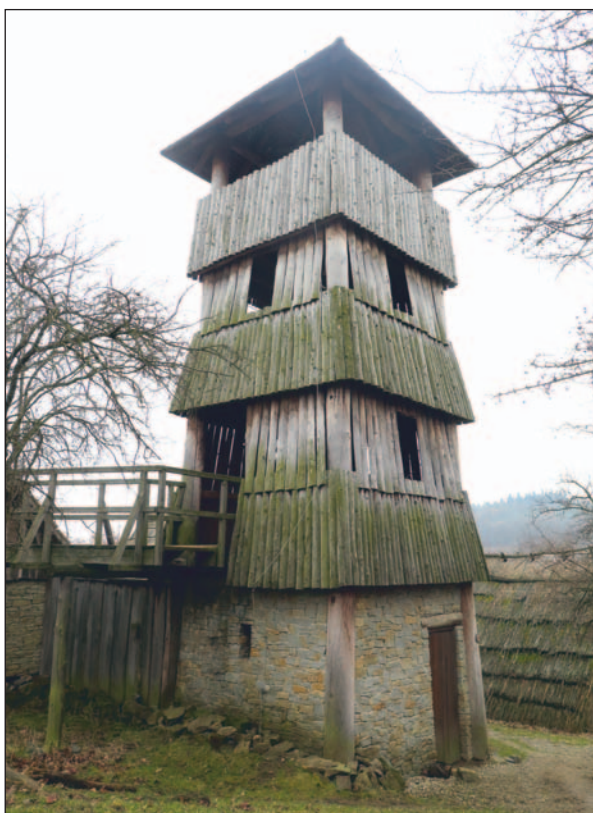
Fig. 12. Modrá. The watchtower with stone foundations and wooden constructions made of red spruce.
