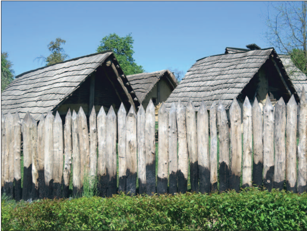
Fig. 10. Modrá. A palisade wall surrounding the archaeological open-air museum with well charred oak poles embedded in crushed stones.
